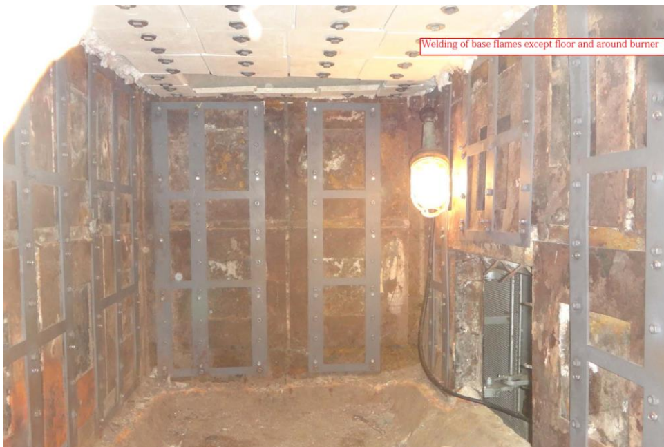
Mounting bolts and installation of ceramic wool
